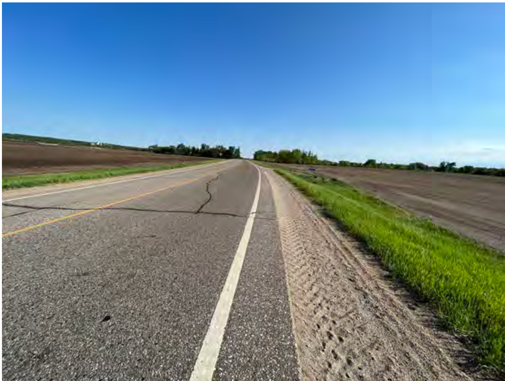
Looking north down County 5
