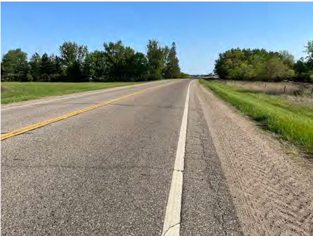
Looking north down County 5
