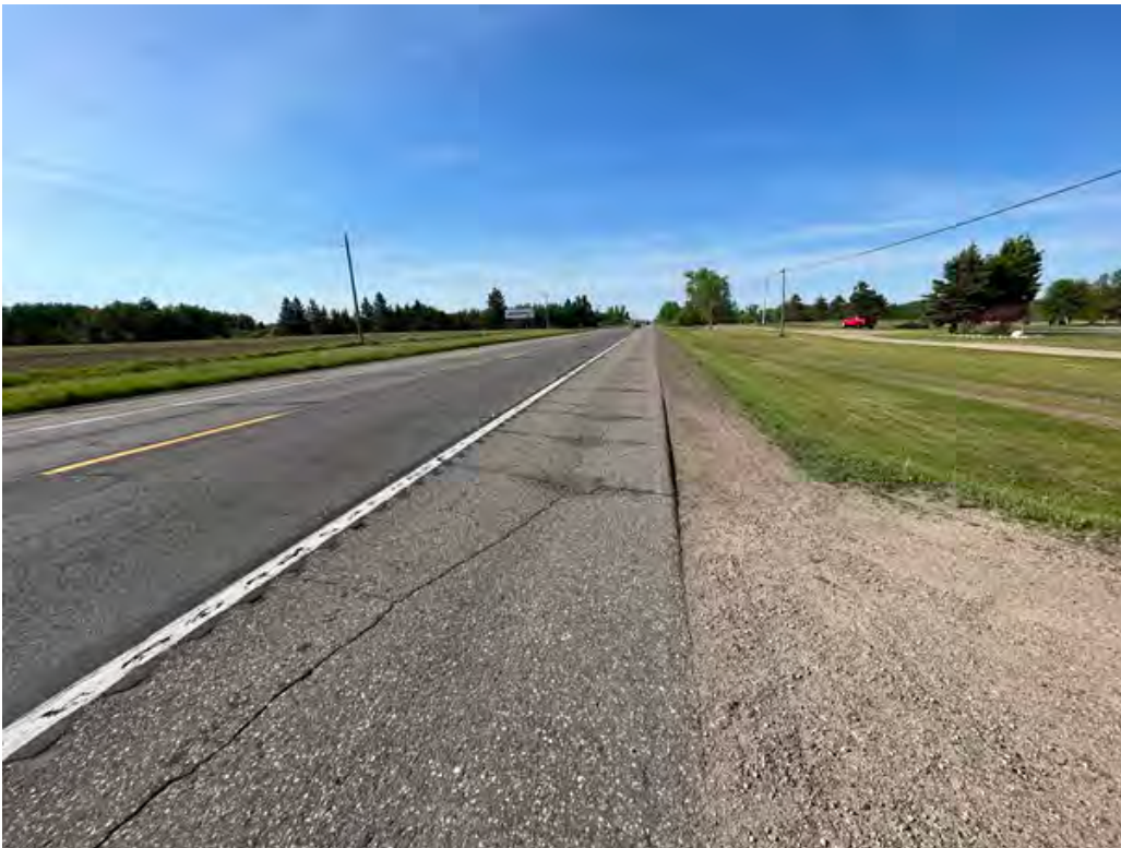
Looking south down US 71
