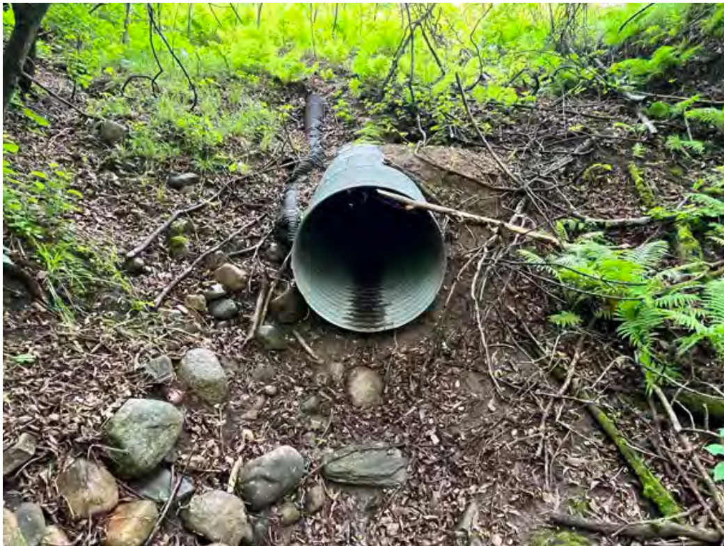
Culvert outlet on the west side of Dunlin Road
