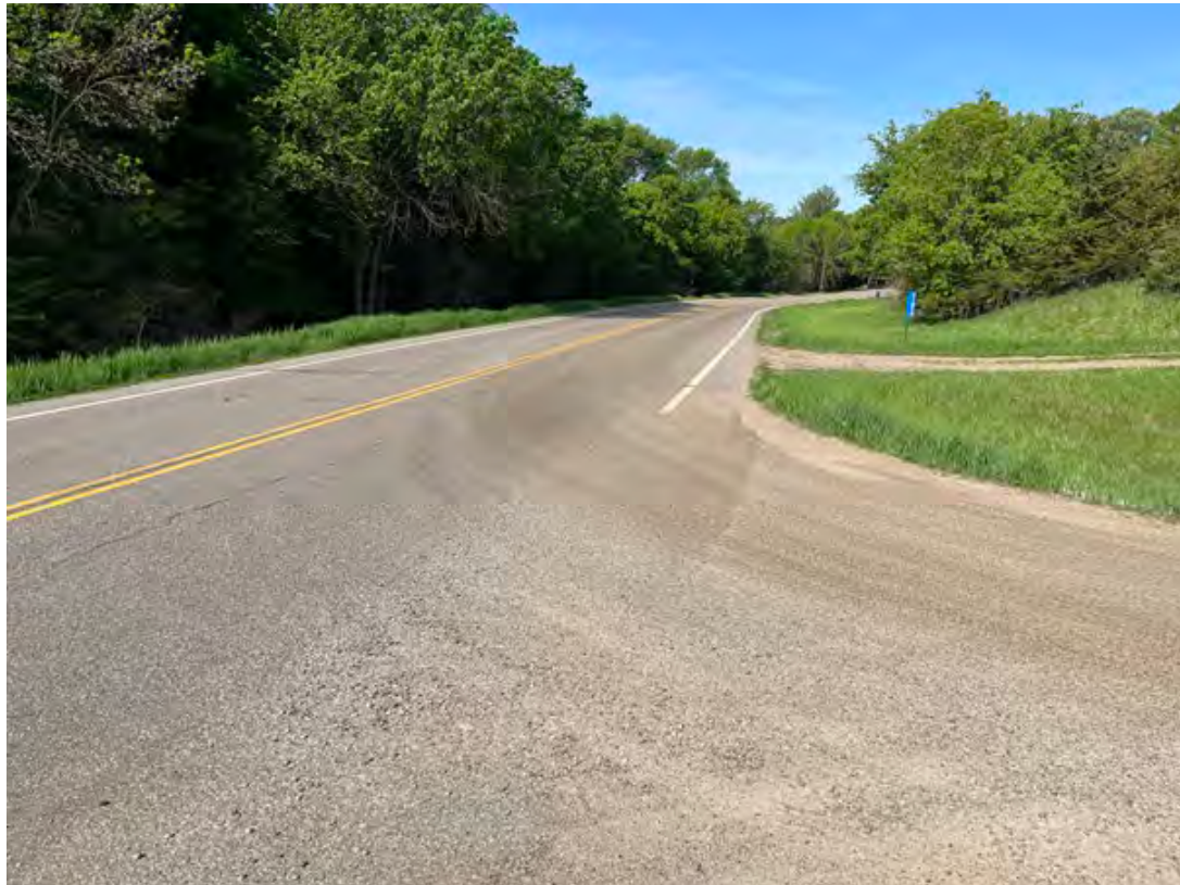
Looking west from the intersection of Dunlin Road and County 13
