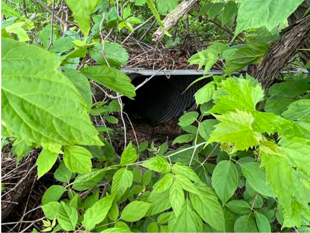
Culvert inlet on the east side of Dunlin Road
